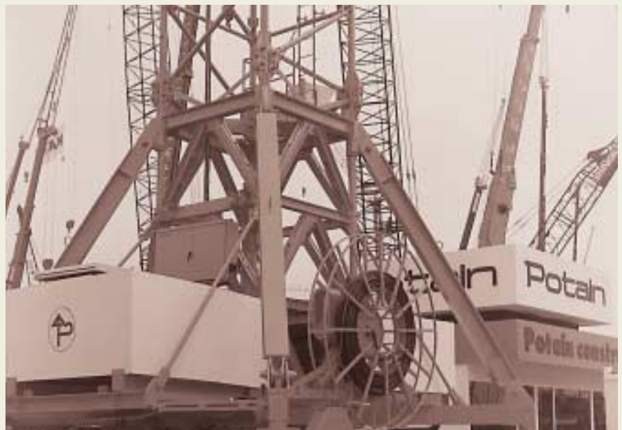
Potain tower crane - 1966.
