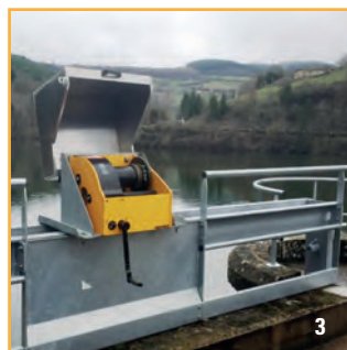
3. Valve lifting.
