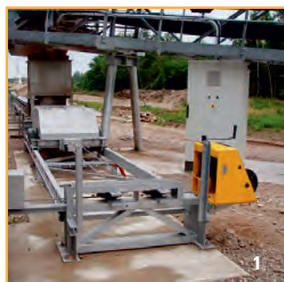
1. Tautening conveyor belts.
